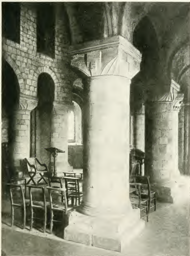
TOWER OF LONDON Chapel of St John, in the White Tower
