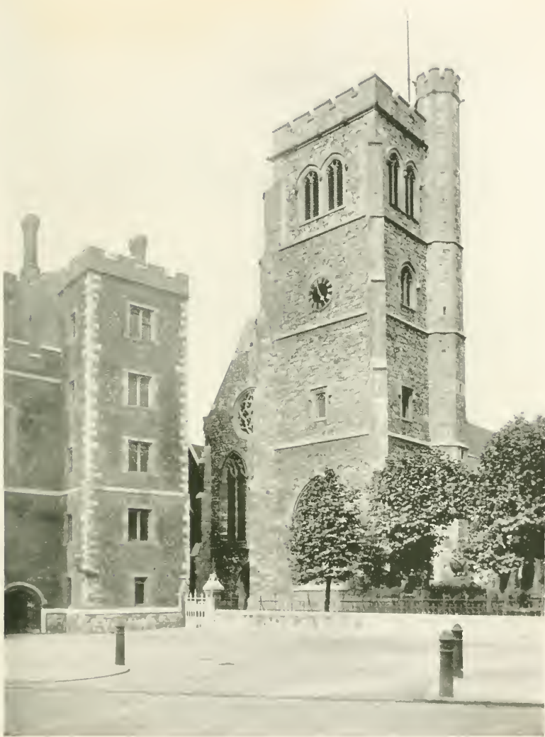
LAMBETH CHURCH AND PALACE GATE
